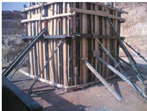
Figure 1. Shuttering for cube.
