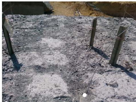
Figure 3. Top view of a cube showing triangular concrete rods. White circle indicates the borehole.
